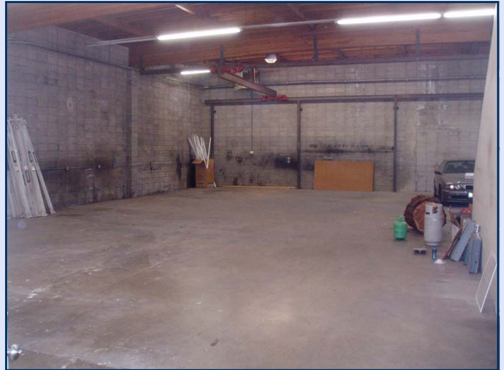
WAREHOUSE WITH CRANE
