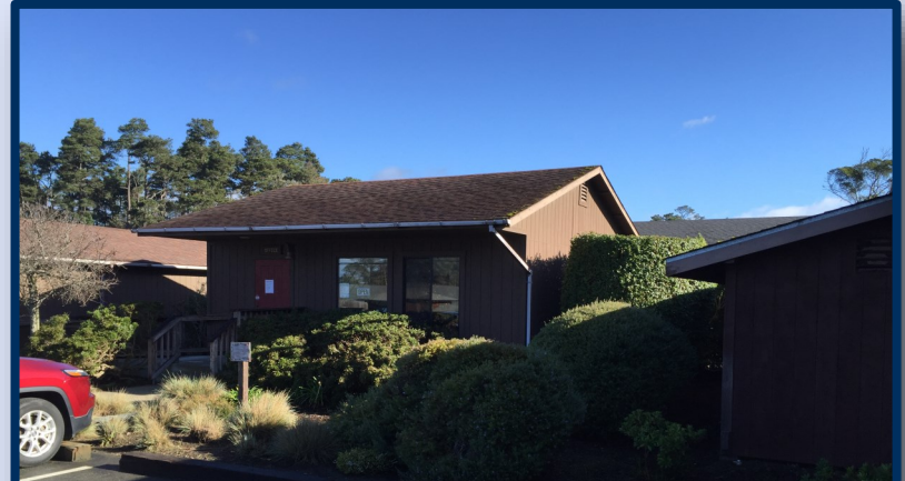
Hopper Dairy Office
