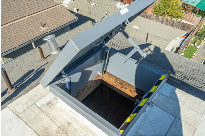
New roof with accessible hatch access
